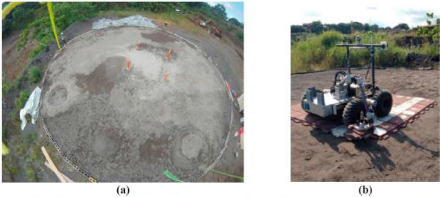
Fig. 6. Proof of concept of the robotic construction of a 20-m VTVL landing pad. a) In-situ basalt Moon-scape; b) Paver deployment mechanism (PDM) [94].
