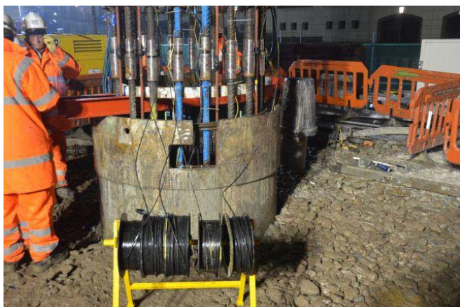
(b) Coiled optical fibres fed into the borehole with the cage
