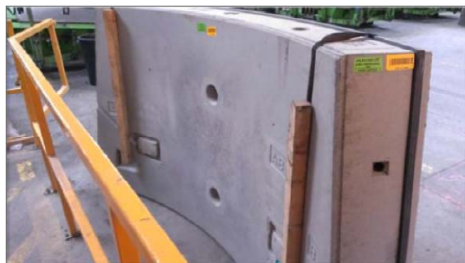
(b) A segment embedded with fibre optic cables
