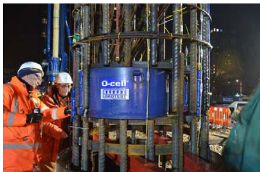
Figure 6. Osterberg cell (O-Cell).
