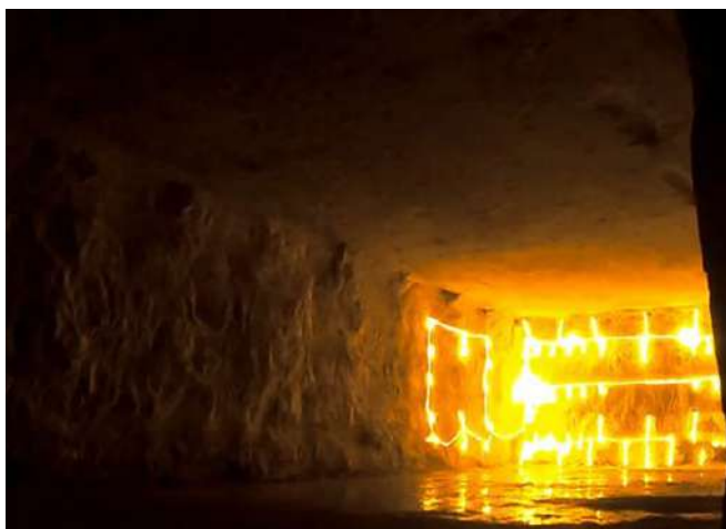
Charged face initiated for a blast round
