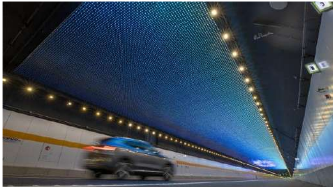
A view of the LED ceiling installed in the 10.79-kilometer tunnel under Lake Taihu.
