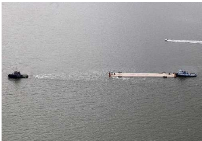
Towing of immersed tube element.
