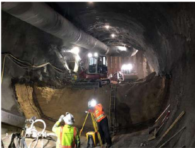
Figure 5. Lower bench excavation completed with lattice girder installed before initial support shotcrete placement; ongoing convergence monitoring with total station.
