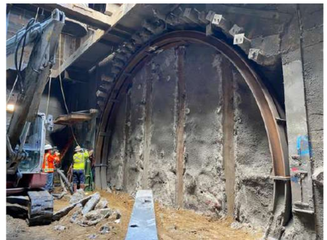
Figure 2. Canopy pipes and a collar beam in place prior to tunnel breakout from starter shaft.
