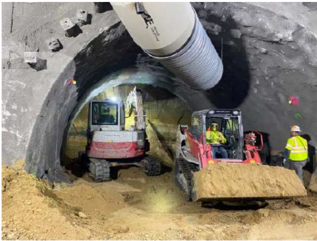
Figure 4. Excavation and mucking of spoils during top heading advance.
