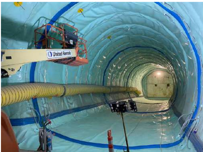
Figure 6. PVC waterproofing membrane installation following completion of initial shotcrete lining throughout entire tunnel cross section.
