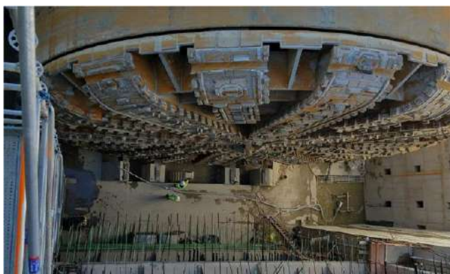
Figure 1. Alaskan Way Viaduct Replacement tunnel: 57.5-ft-diameter TBM cutterhead in the exit shaft.
