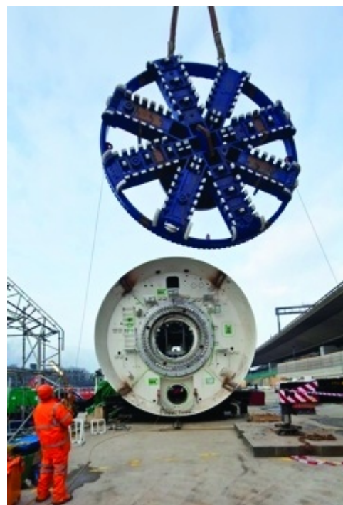
The 7.1m diameter cutting head is lowered into place on the front of the tunnel boring machine
